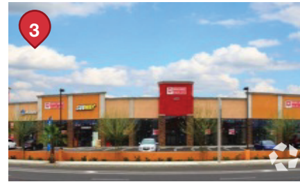
6201 Whittier Blvd • Los Angeles
