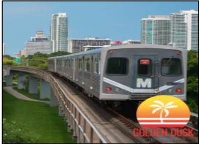
The Metrorail : A 23 station, 25-mile elevated rapid transit system which connects Brickell to Miami International Airport, Coral Gables, Downtown, and the various communities in all of Miami-Dade County.
