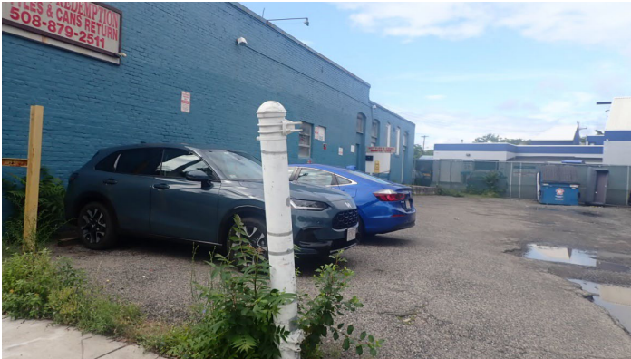
Side access and parking
