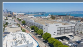
American Industrial Center
