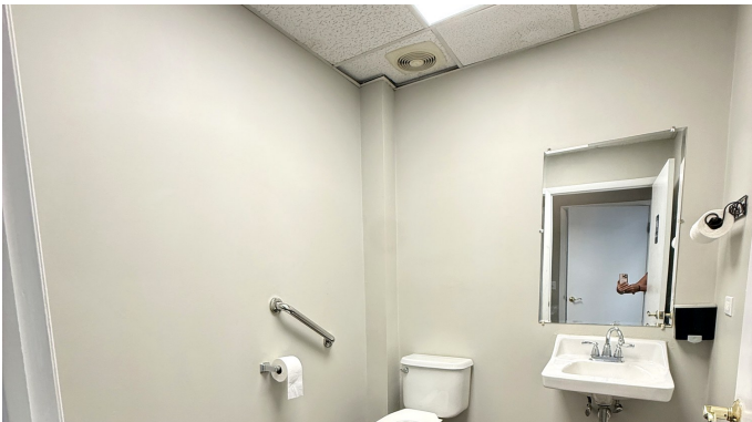
ADA RESTROOM WITH GRAB BAR
