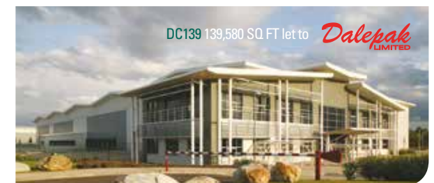
139,580 SQ FT DISTRIBUTION CENTRE AT PROLOGIS PARK PINEHAM
