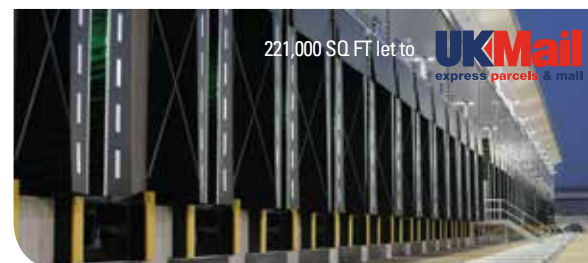
221,000 SQ FT DISTRIBUTION CENTRE AT PROLOGIS PARK RYTON
