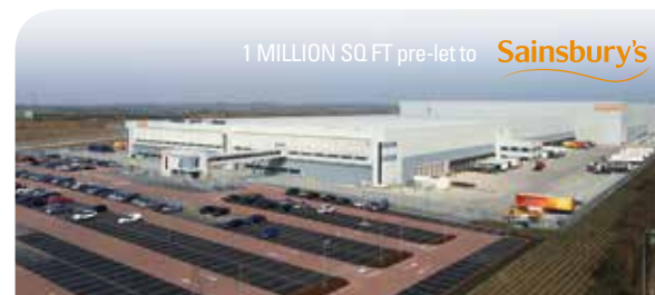
1 MILLION SQ FT DISTRIBUTION CENTRE AT PROLOGIS RFI DIRFT
