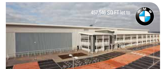
457,546 SQ FT REGIONAL DISTRIBUTION CENTRE AT PROLOGIS PARK PINEHAM
