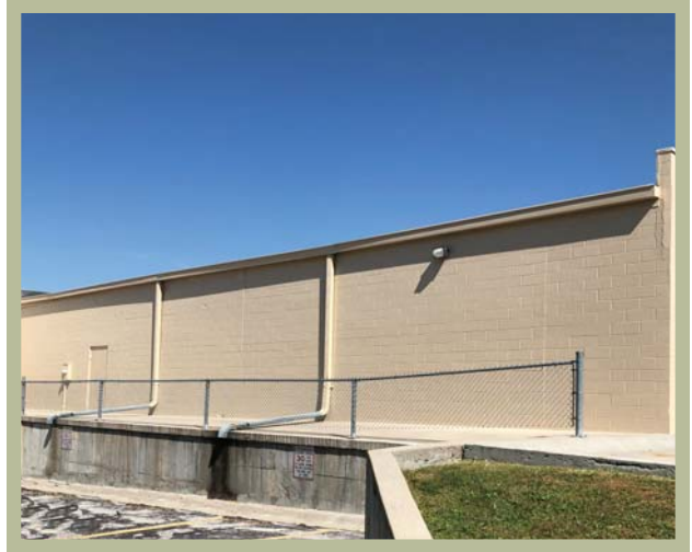
Exterior Photo: Rear Entrance
