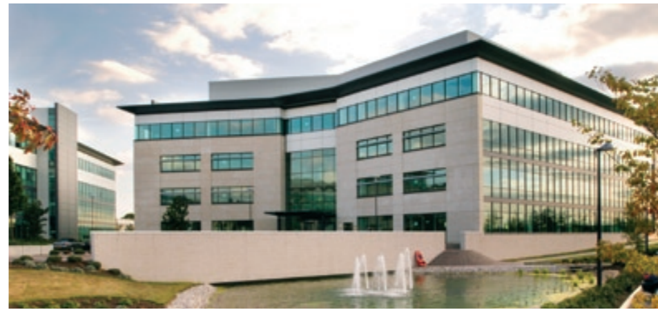
450,000 sq.ft. HQ campus built-to-suit for T-Mobile, Hatfield Business Park.
