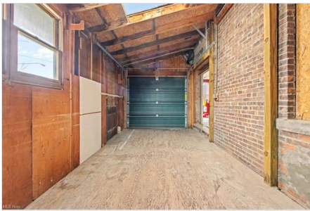
View of garage
