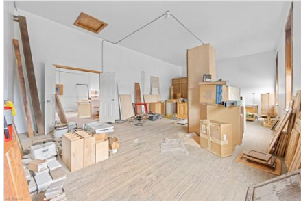
View of miscellaneous room
