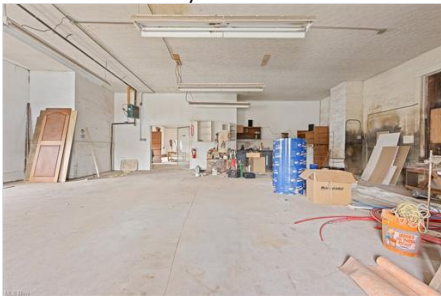
Garage featuring a garage door opener
