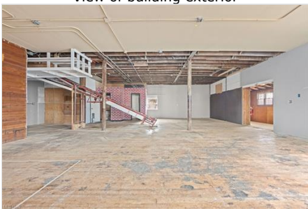
Basement with wood walls
