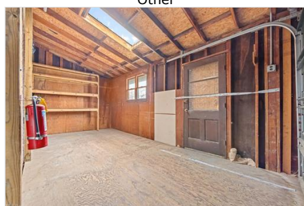
View of storage room
