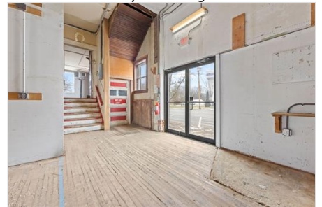
View of lobby
