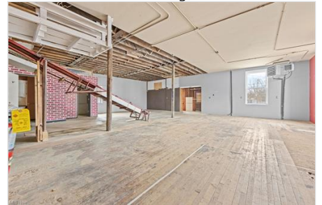
Basement featuring a wall unit AC
