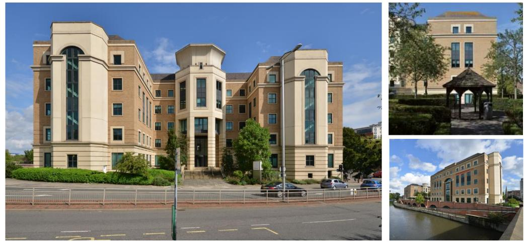
The Alpha Building forms part of 121 Kings Road, developed by Kumagali Gumi UK Ltd, reaching practical completion in January 1993. The building is arranged around an H shaped floor plate and comprises 68,438 sq ft NIA of office accommodation over ground and four upper floors. The property is of reinforced concrete framed construction, with brick and stone elevations under a part pitched slate clad roof.
