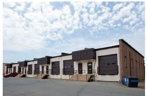
Loading Dock Entrances
