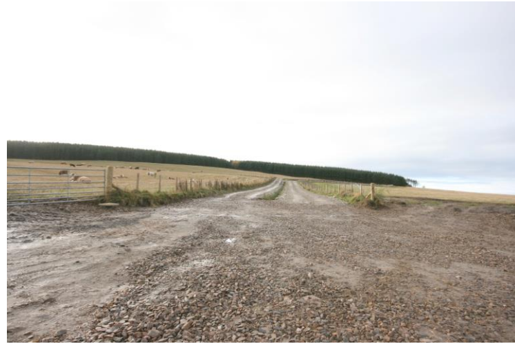
A hardcore road has been laid giving access to the plot
