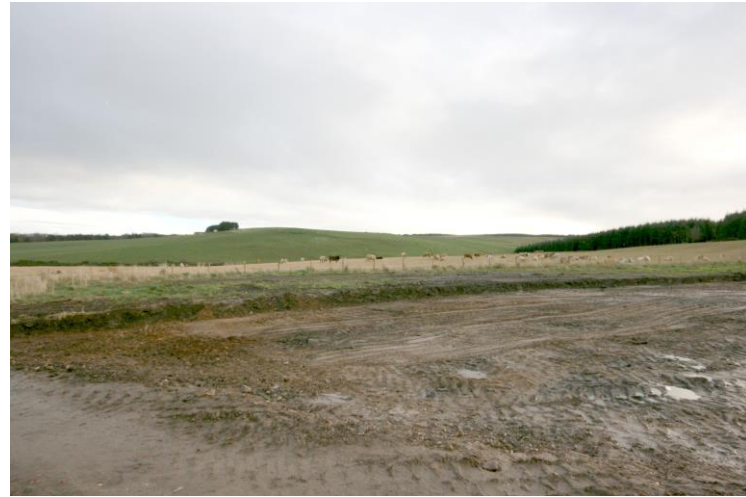
The site has been cleared
