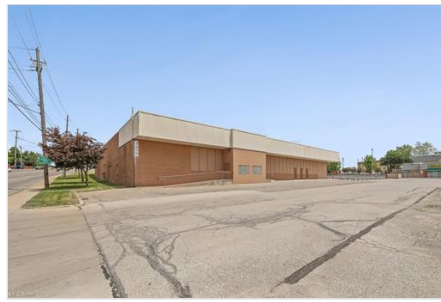
Front of Structure
