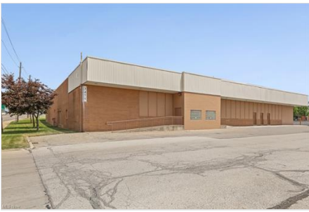
Front of Structure
