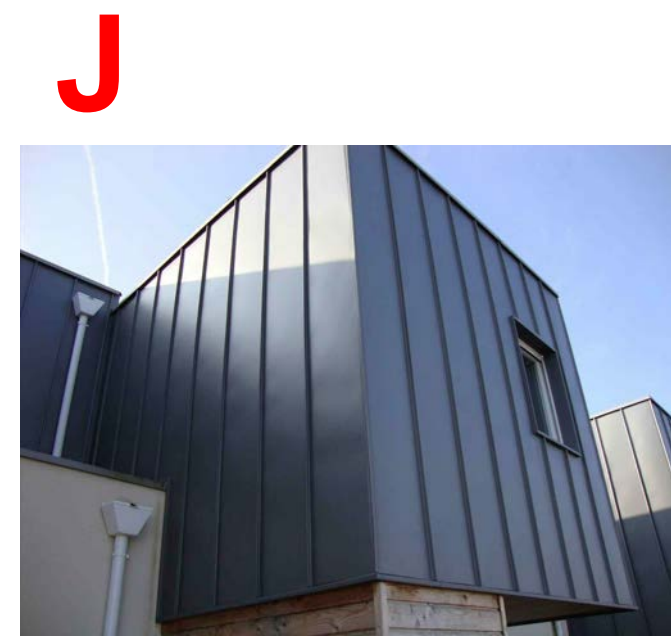
J VERTICLE METAL SIDING - OCCURING ON NORTH AND SOUTH ELEVATIONS
