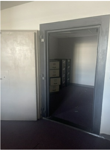
Interior View - Vault/Storage
