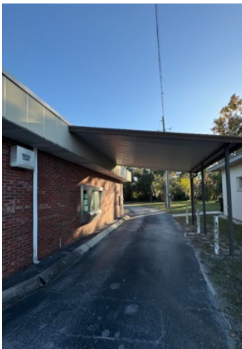
Interior View - Canopy
