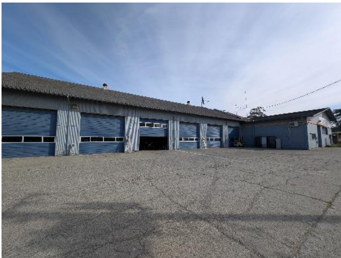
TYPICAL EXTERIOR VIEW
