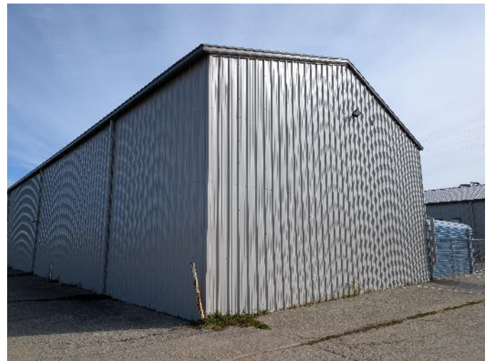
TYPICAL EXTERIOR VIEW
