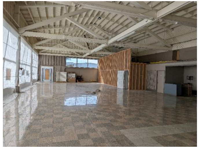
TYPICAL INTERIOR VIEW
