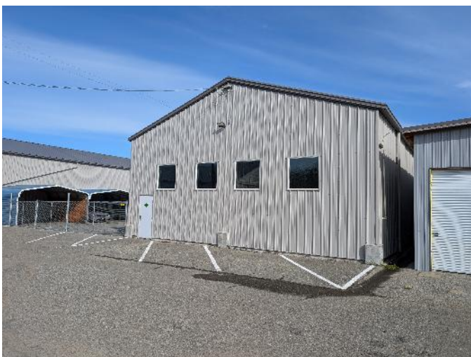
TYPICAL EXTERIOR VIEW
