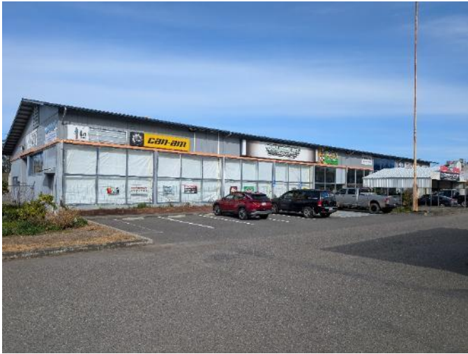
TYPICAL EXTERIOR VIEW
