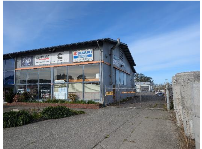
TYPICAL EXTERIOR VIEW
