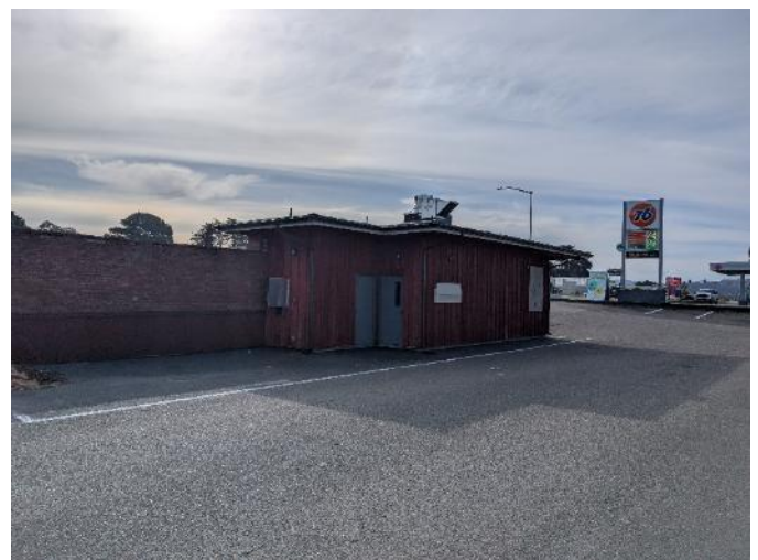
TYPICAL EXTERIOR VIEW
