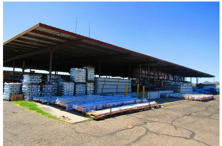
Canopy Area (note—has truck well loading)
