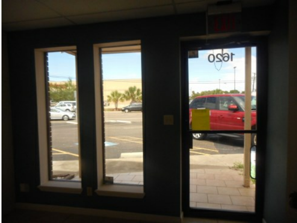
Interior Photo - Front Entrance
