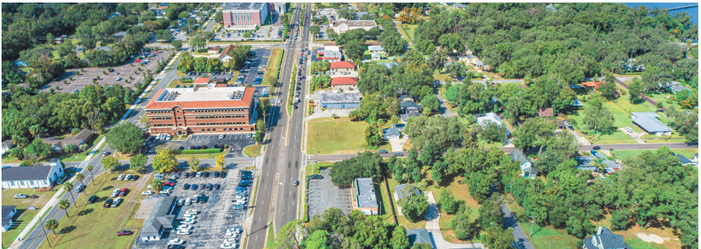
Regional aerial showing U.S. 17, county facilities, surrounding development and the St. Johns River.
