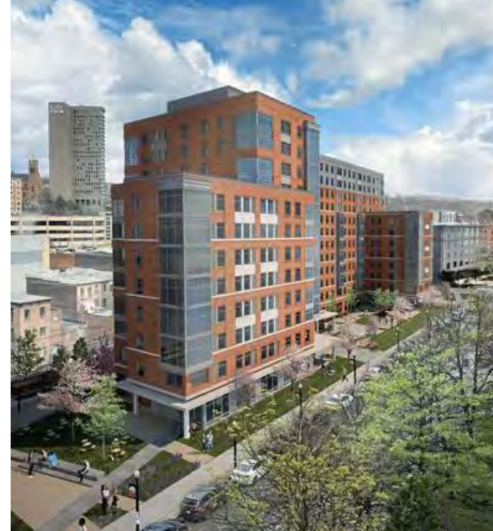
11-story student apartment building on Forbes Avenue
