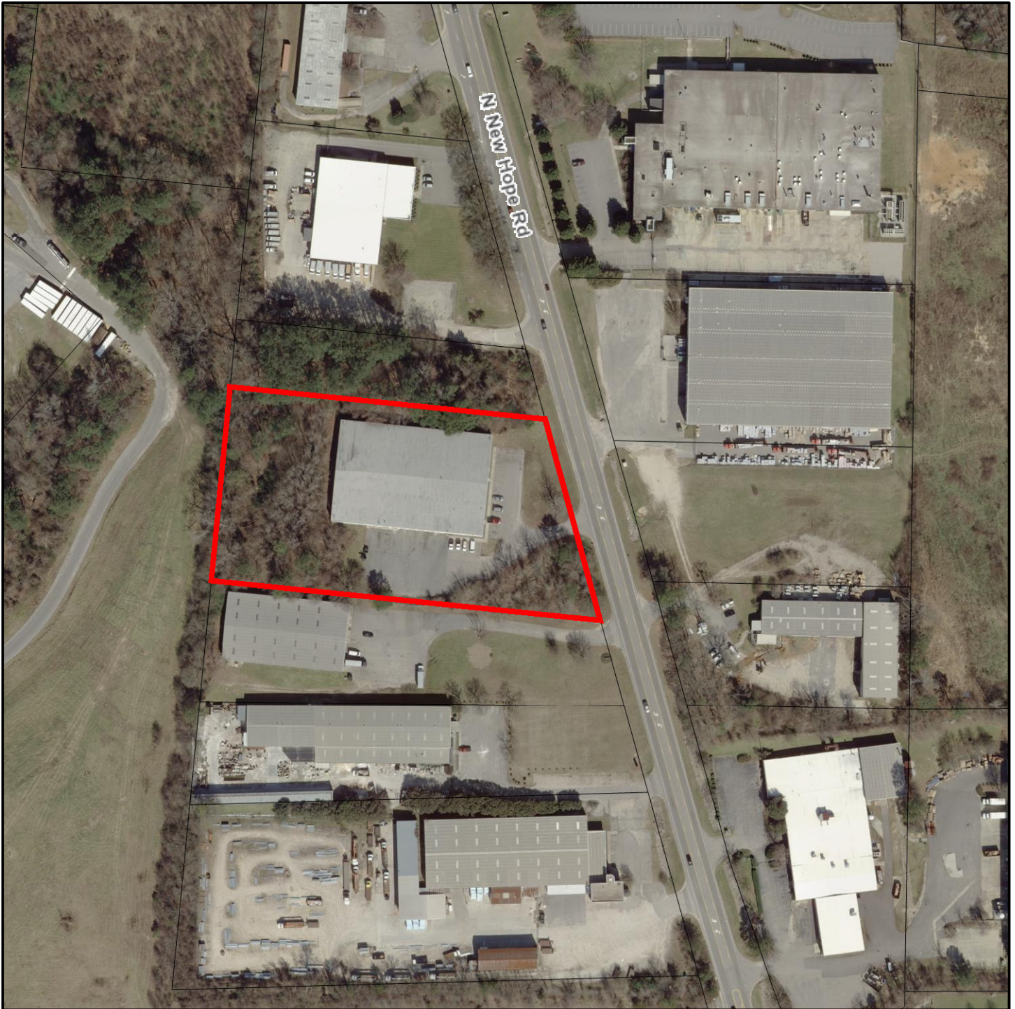
1115 N New Hope Road Aerial
