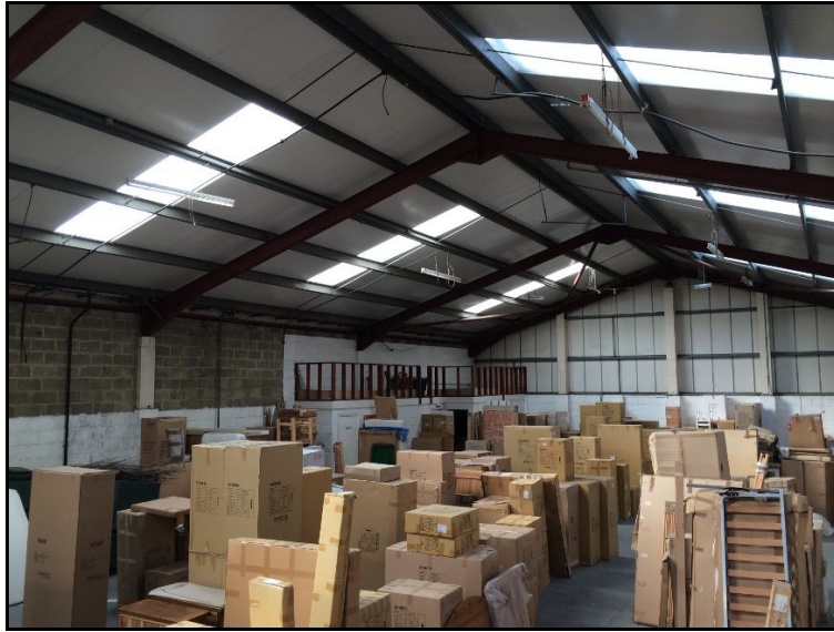
The warehouse of Unit 6
