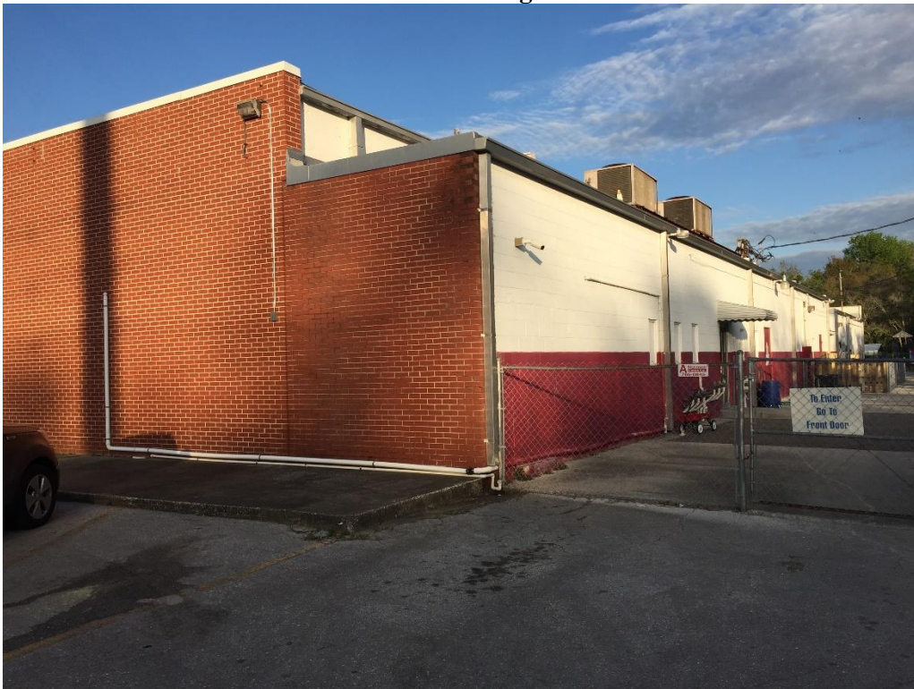
West Side and Rear of Building One
