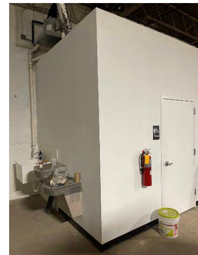
Inside View of Bathroom
