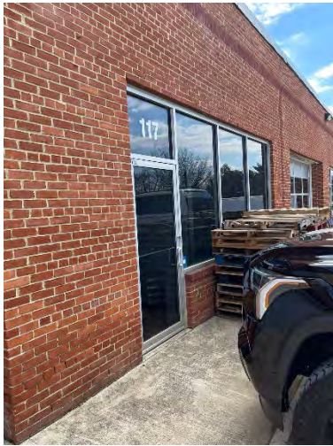
View of Entrance Door
