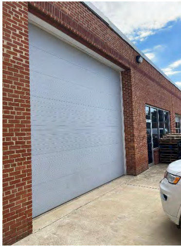
View of Drive-In Door
