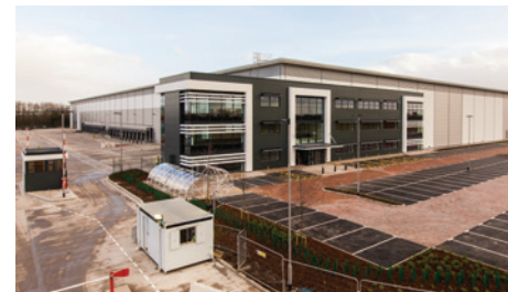
Amazon 277,089 sq ft industrial unit, Airport City, Manchester.
