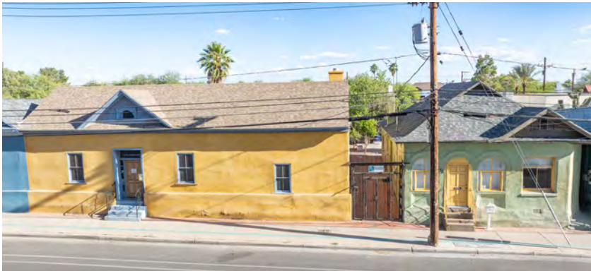
Street View along Cushing Street
