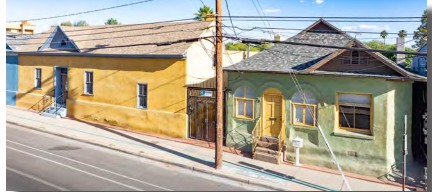
Street View along Cushing Street
