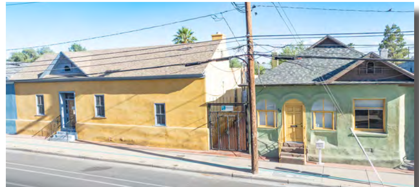
Street View along Cushing Street
