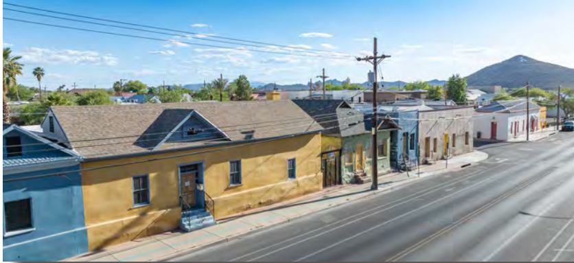
Street View along Cushing Street
