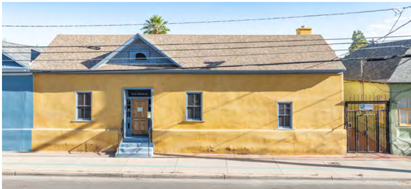
Street View along Cushing Street
