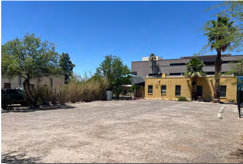
South Parking Lot #1 Looking North - Back of 70 W Cushing St.
