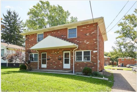
Front of Structure
