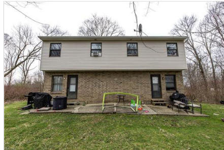
Back of Structure
