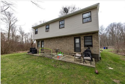
Back of Structure
