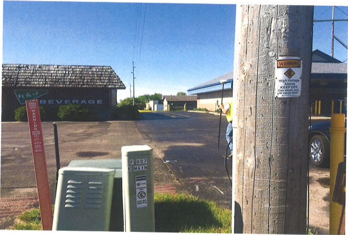
EAST PROPERTY BOUNDARY, LOOKING SOUTH
