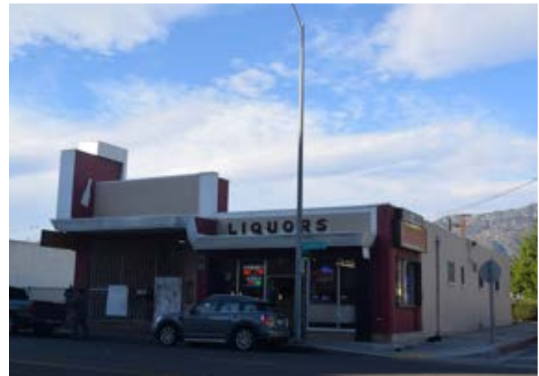
Foothill Liquor Building, 2547 E Foothill Blvd.
