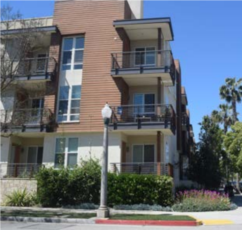
Private Open Space (Balconies).
