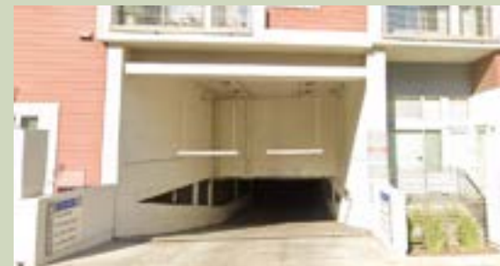
Garage entrance without screening or façade integration.
