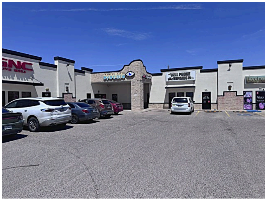
Entry tower and lighted signage bands at the center's midpoint
