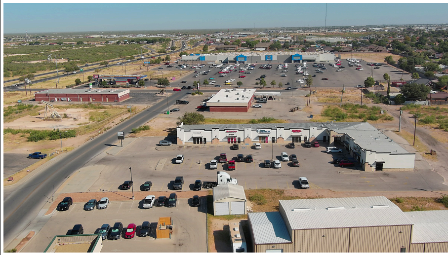
Looking northwest — the center in the foreground, Walmart Supercenter and NW Loop 338 beyond
