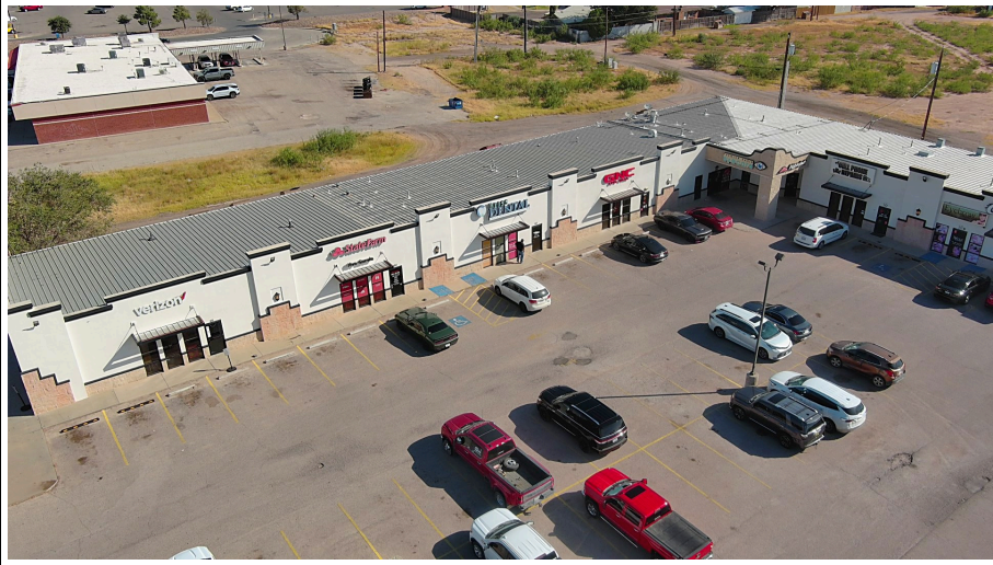
Linda Retail Center — ±55,283 SF site, 170 parking spaces
