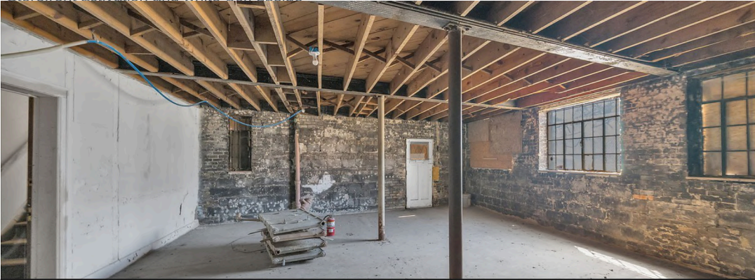
EXISTING COMMERCIAL SHELL / EXPOSED STRUCTURE
