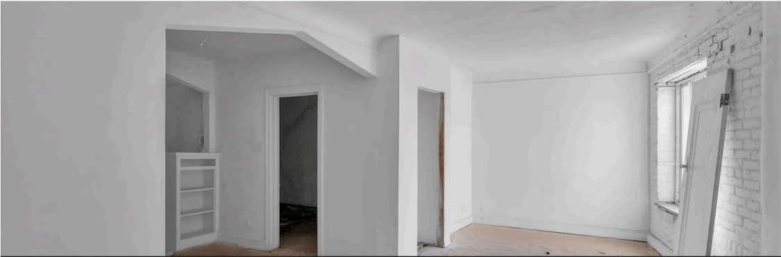
RESIDENTIAL UNIT - EXISTING RENOVATION CONDITION
