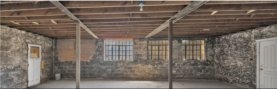
COMMERCIAL SPACE - EXISTING WHITE-BOX SHELL
