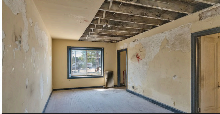
EXISTING CONDITION UNIT
