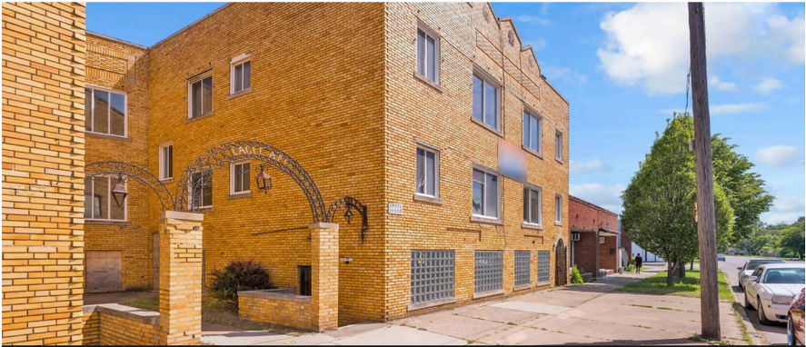
FRONT FACADE / MACK AVENUE FRONTAGE
