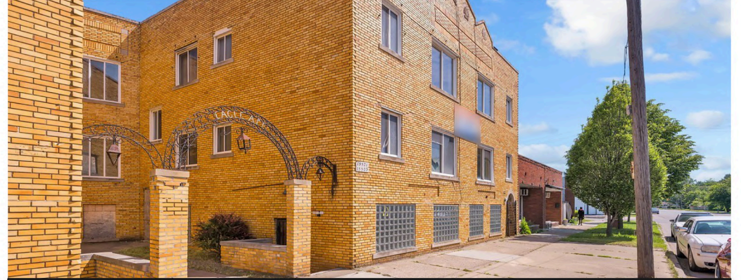
MACK AVENUE FACADE
