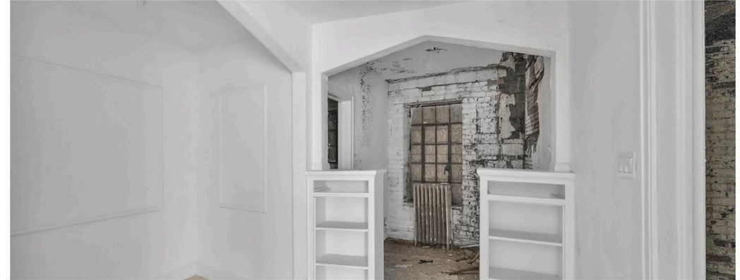
LARGE UNIT LAYOUT / RENOVATION PROGRESS
