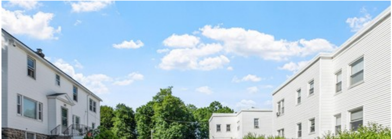
Ureco Terrace: 3 Ureco Terrace on left, 2 Ureco Terrace and 827 Pleasant Street on right
