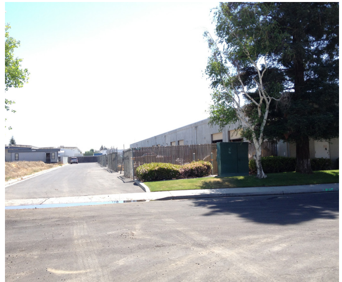
View of Back of Building (Yard)
