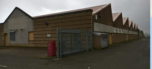
The subjects comprise a single storey detached industrial unit of brickwork construction partially roughcast rendered externally and facing blockwork externally in part. The roof is predominantly of pitched design with a series of six pitches to the main building clad in profile metal sheeting. The building is surrounded by an enclosed tarmac surfaced yard area with significant yard/ car parking facilities serving the building.
