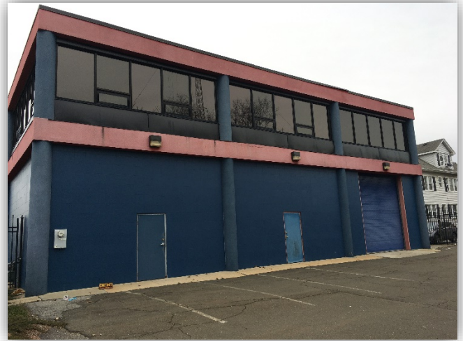
Rear of Building
