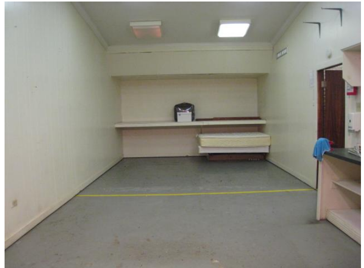
Large open room at rear of bldg.
