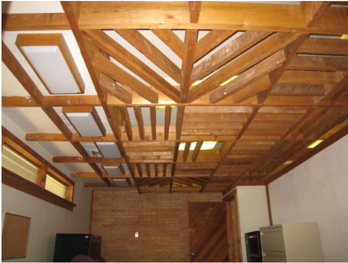
Ceiling treatment in office- Is removable
