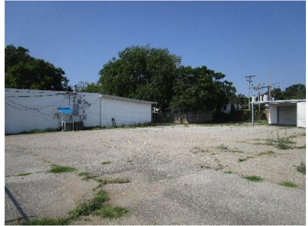
Photo #2 View of the site as seen from the northeast corner of the site.
