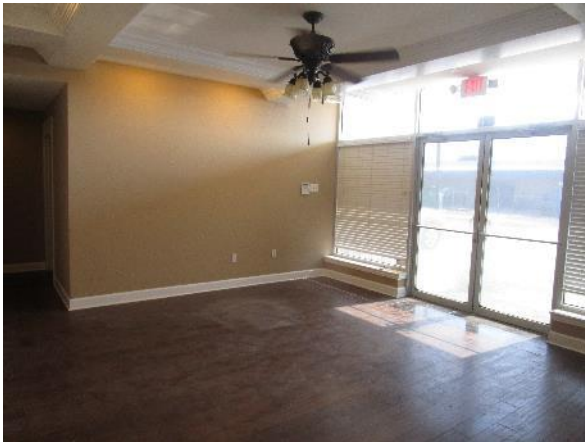
Photo #3 Typical view of the front entrance area of the office building.
