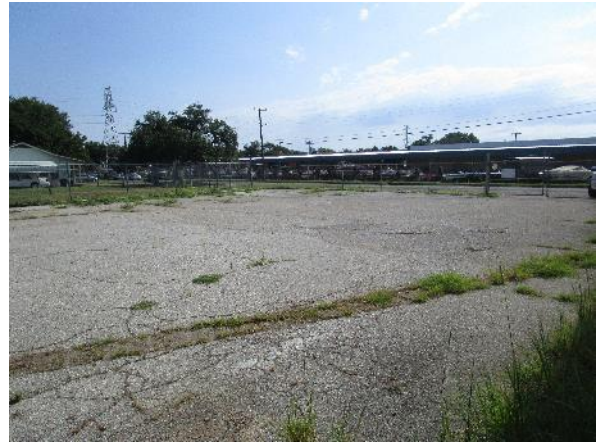
Photo #10 View of the asphalt-paved parking area on the northern portion of the site.
