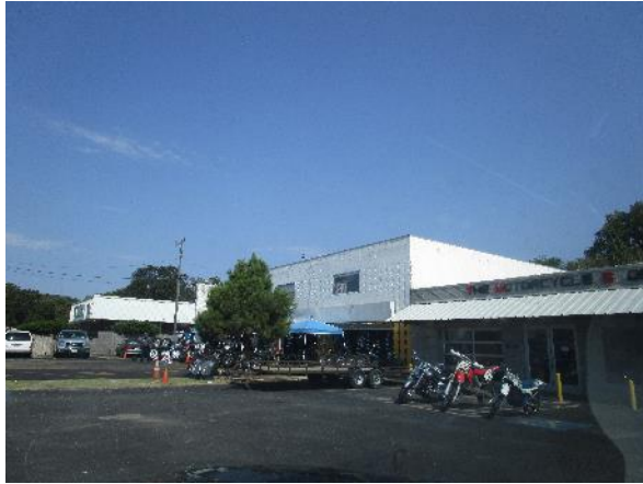
Photo #13 View of the south adjoining Motor Cycle Shop, A&A Tire & Wheels, and Cody Air Conditioning and Heating.
