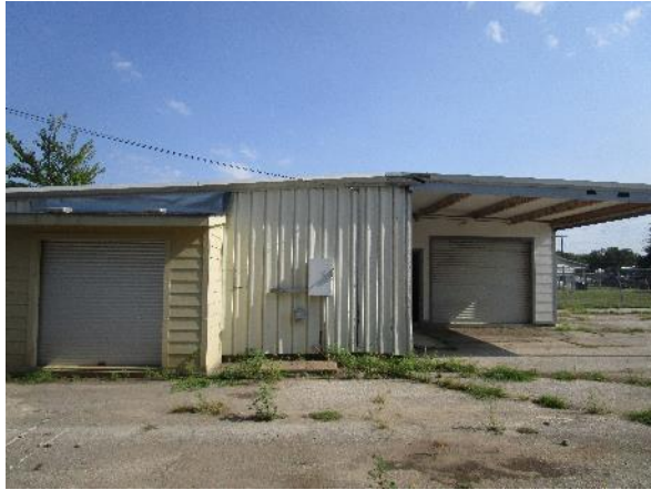
Photo #7 View of the exterior of the storage/warehouse building.
