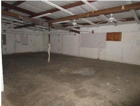
Photo #9 View of the equipment storage portion of the storage/warehouse building.
