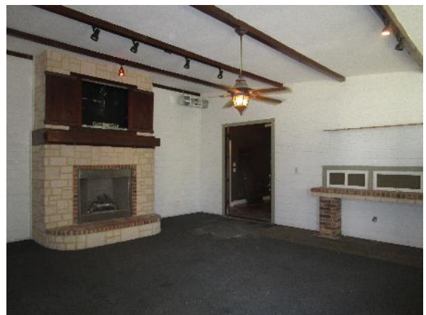
Photo #6 Typical view of the light fixture room located in the western portion of the office building.
