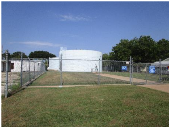
Photo #11 View of the City of Hurst Water Utilities Division Pump Station located to the north and west of the site.
