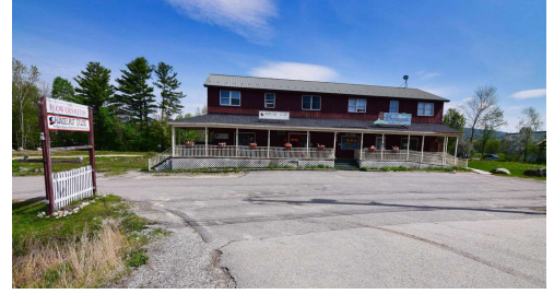
Curb cut on Tenney
