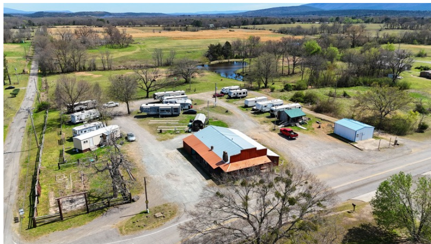
AERIAL — RV SITES & COMMERCIAL BUILDING
