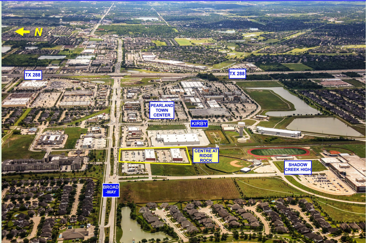
LOOKING EAST TOWARD MAJOR TX 288 / BROADWAY INTERCHANGE
