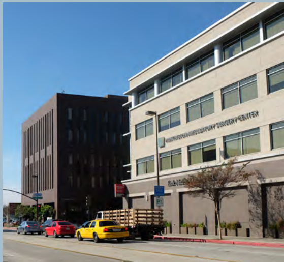
Medical office uses at Fair Oaks Ave and Congress St include 4-5 story buildings, several of which include non-transparent ground floors
