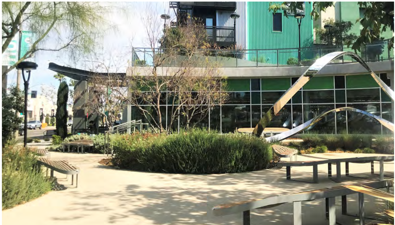
A publicly accessible corner plaza creates a space to gather or rest, including amenities such as seating, landscaping, shade trees, and public art
