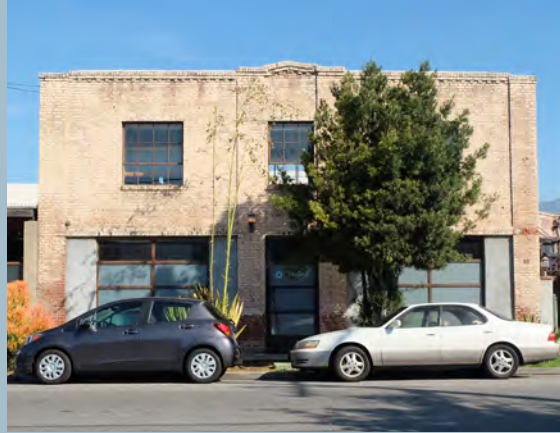
Brick warehouse building being adaptively reused in the SFOSP area
