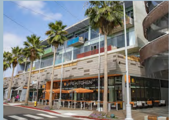
Integrated medical clinic in mixed use development with large second floor terrace that connects activity to the ground floor and creates an amenity for patients, employees, and visitors.
