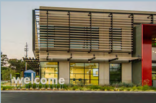
Adaptive reuse medical office with aluminum louvers which mitigates solar heat and glare while also creating privacy
