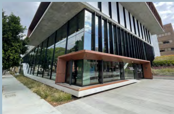
Ground floor landscaping surrounds a primary entrance and sets the building back from the street, protecting street trees
