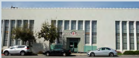
Royal Laundry Building at 443 S Raymond Ave (built 1915)
