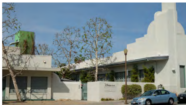
Historically designated Art Deco style building along Raymond Ave currently occupied by a software company
