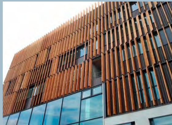
Medical research center with contemporary architectural features including wood screen and glazed façade
