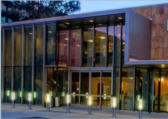
Medical office with a primary entrance from the street and a transparent ground floor with patient registration and wayfinding
