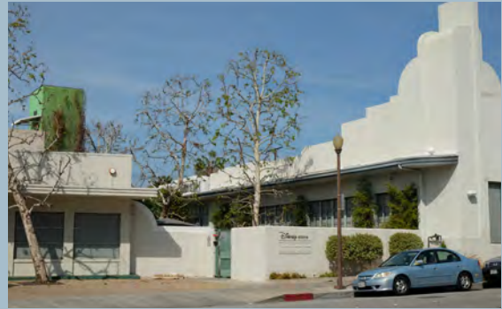
Historically designated Royal Laundry building along Raymond Avenue with art deco style and features
