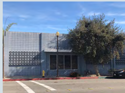
Office building at 650 S Raymond Ave (built 1965)
