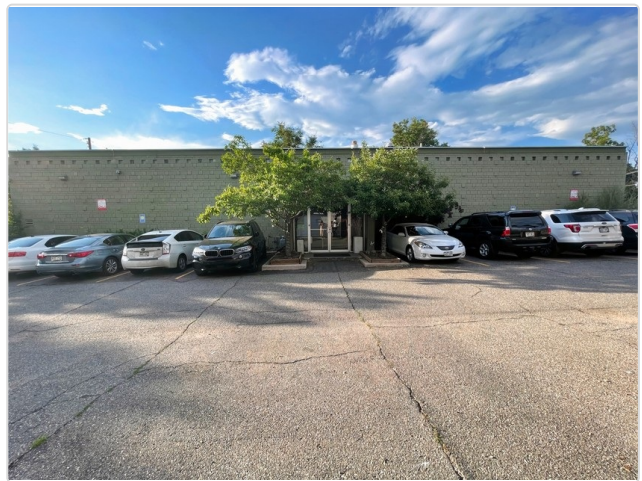
Building Exterior — 520 Cherokee St
