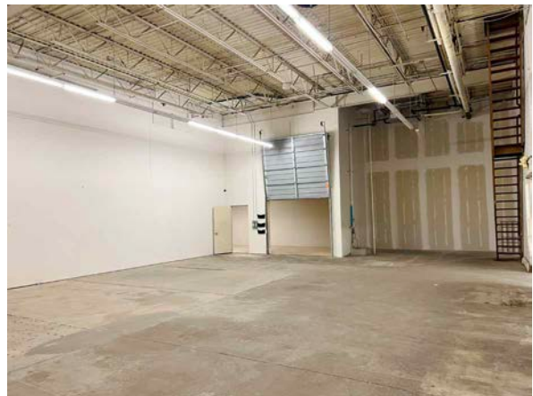
Middle Storage Room
