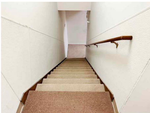
Stair to Upper Level East
