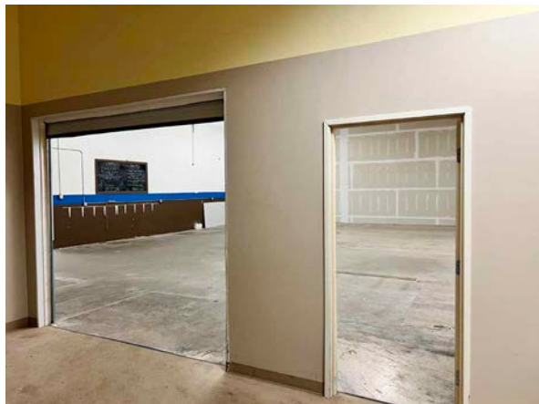
Doors to Middle Storage Room
