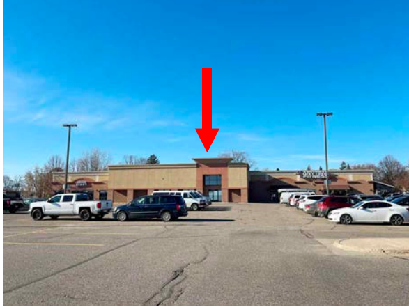
Retail Center Containing Unit 3A
