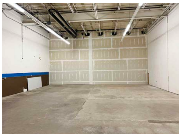
Middle Storage Room
