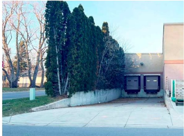
Loading Docks to Back Storage Room
