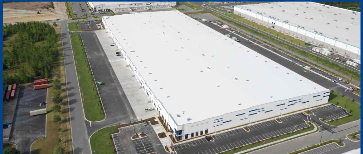
Site aerial taken September 2021
