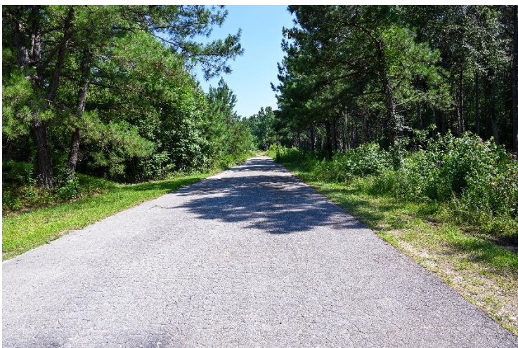
Existing paved drive within the site.
