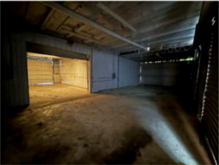
Interior View of Warehouse
