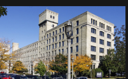
53 THE TANNERY, MILWAUKEE (TIMBERS BUILDINGS)
