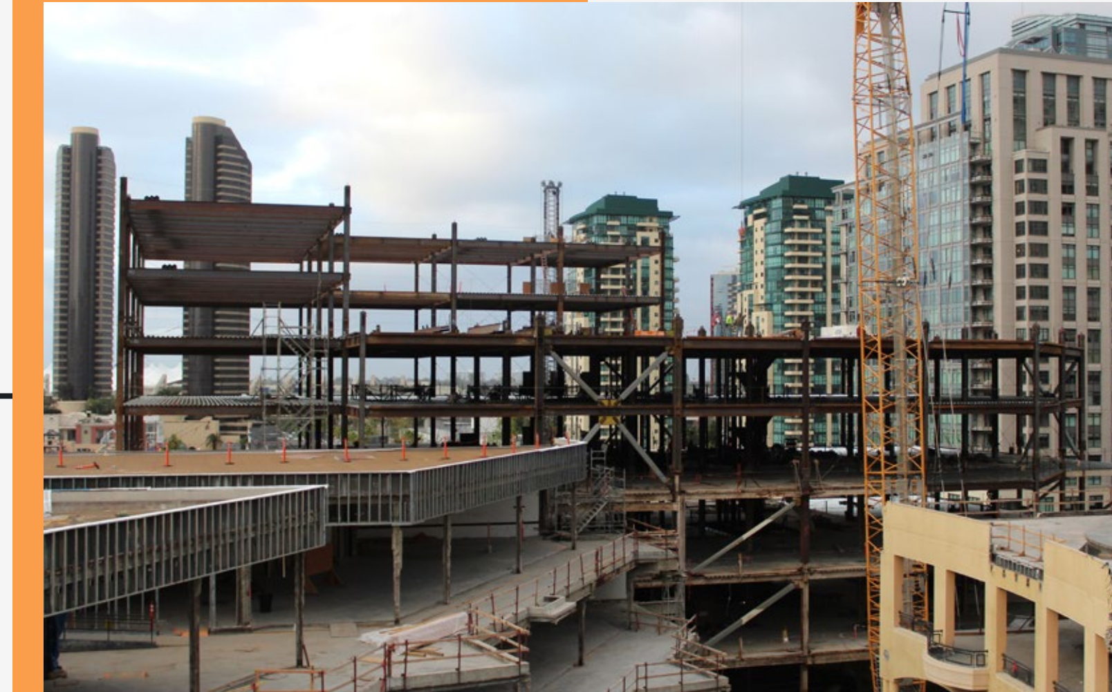
Construction is well underway | Photo taken: March 2021
