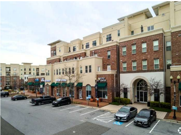
View of Shops at Midtown
